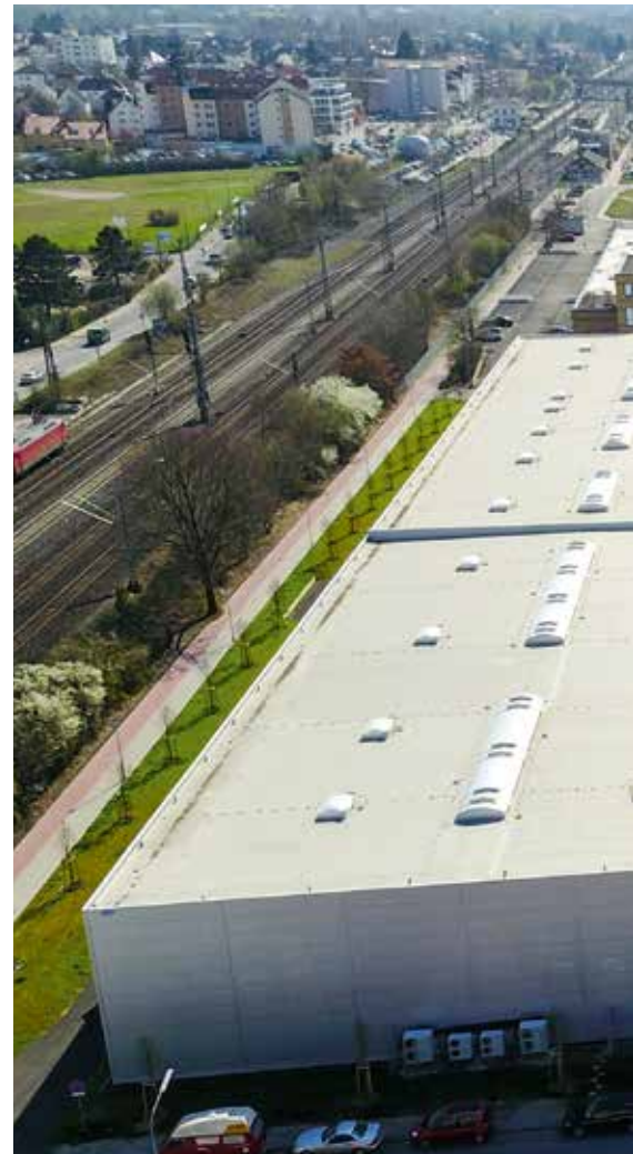
Series production facility in Langen
